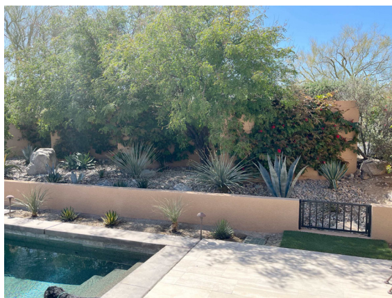
After — Finished Wall
